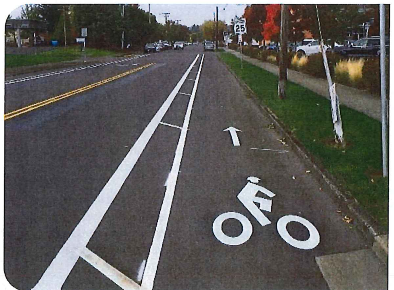
3' buffered on-road bike lane
