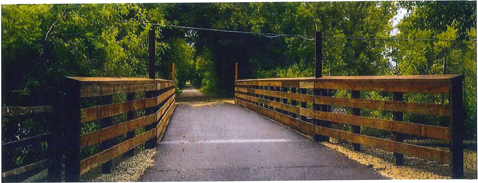
Shared-Use Paved Trail Bridge
