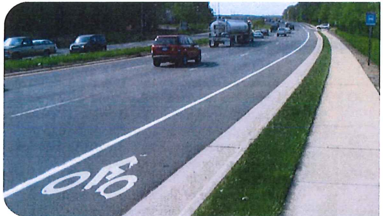
Non-buffered on-road bike lane
